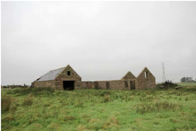
Plot 2, Cowhills Steading extends to approximately 0.67 acre and also includes a paddock extending to an additional acre.
