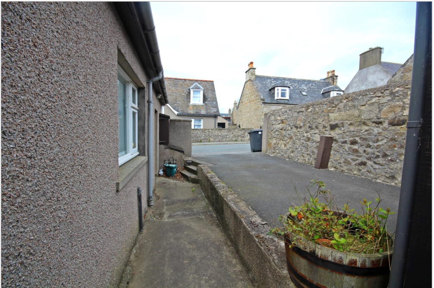
Drive for Off-Road Parking
