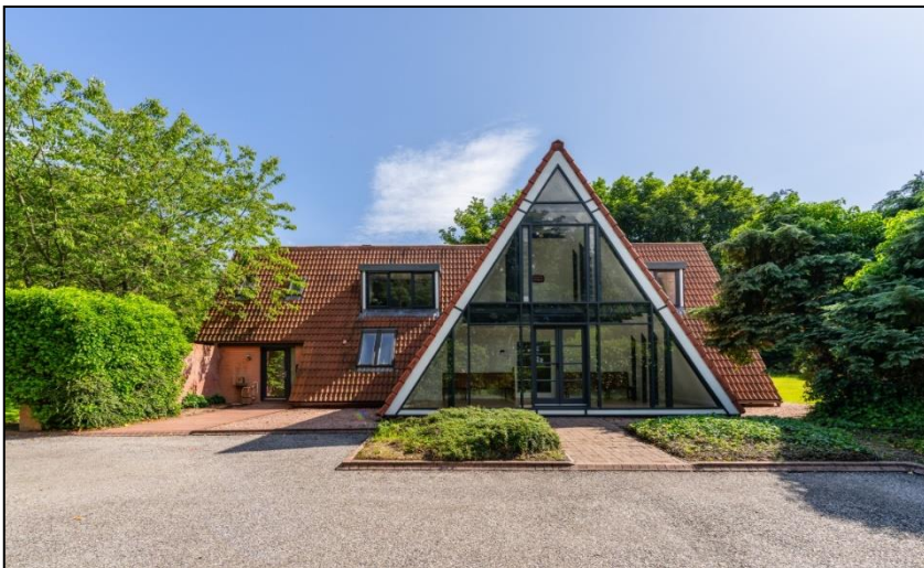
Garage & Front of Property
