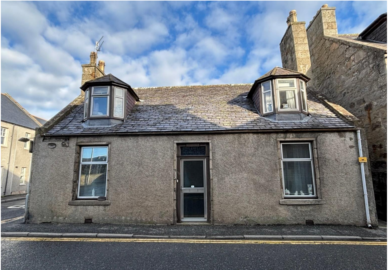
Traditional Stone-Built Detached Dwelling in Central Location
