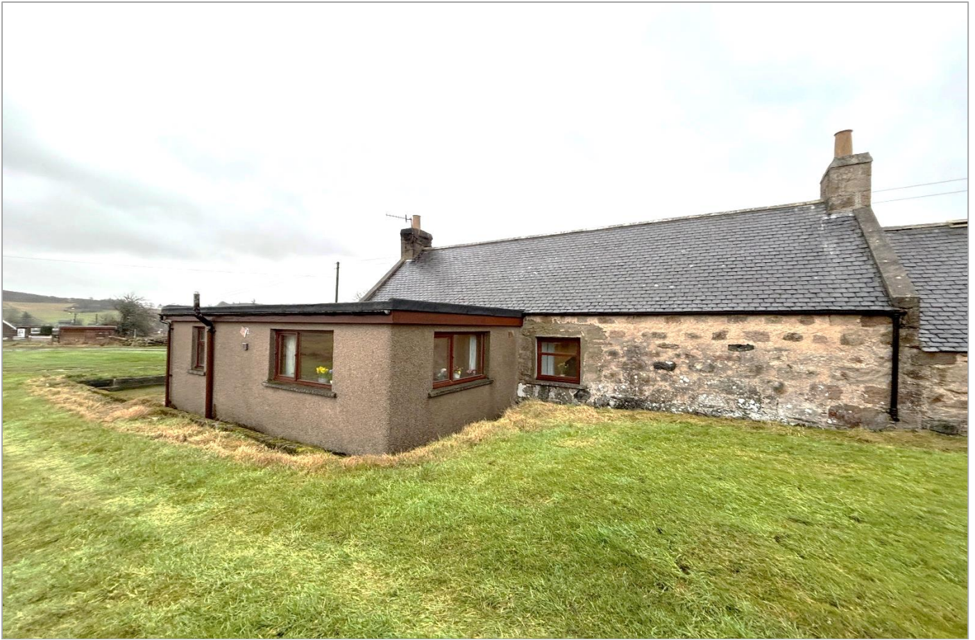
View of Extension to the rear
