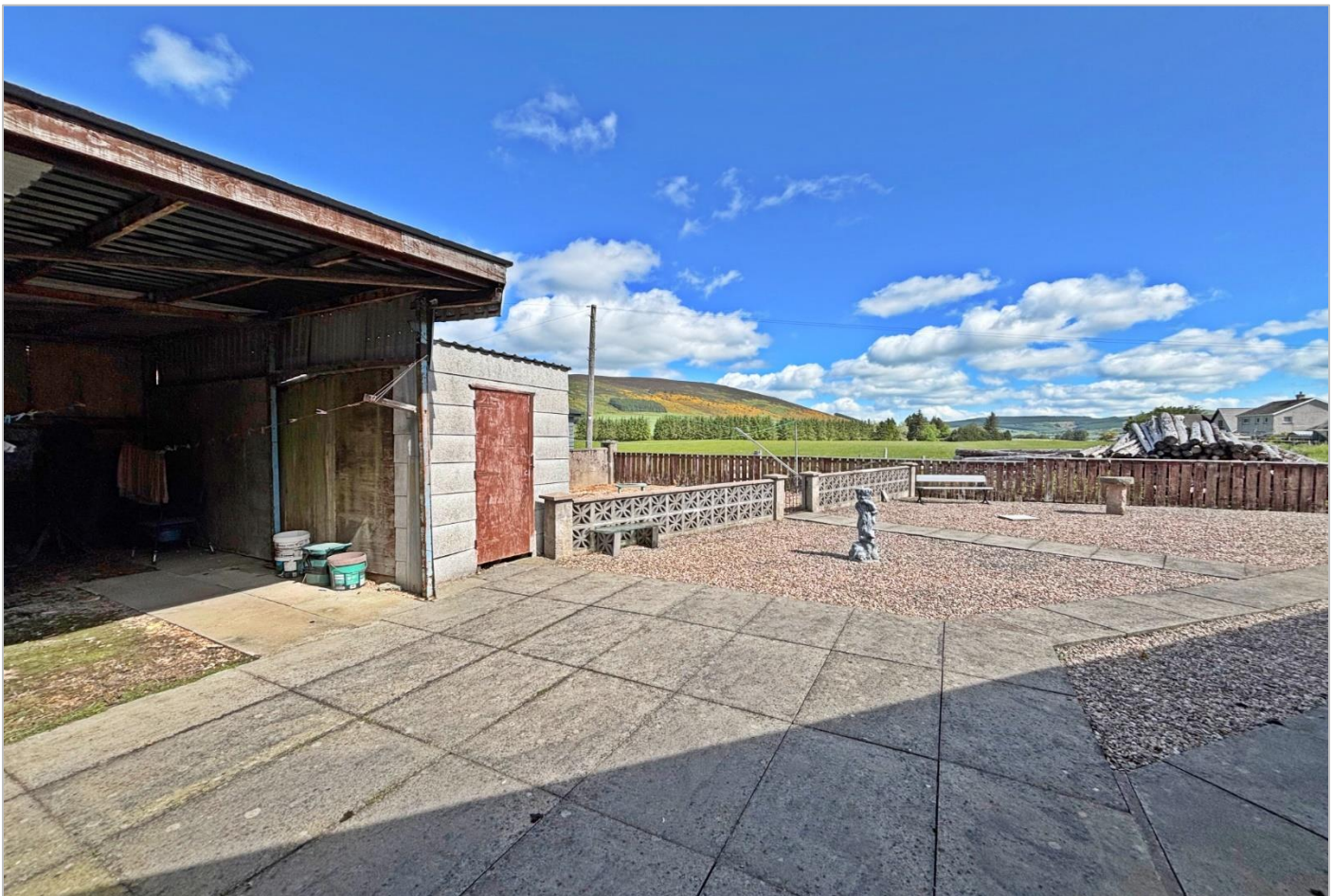
Covered Car/Storage Area to rear
