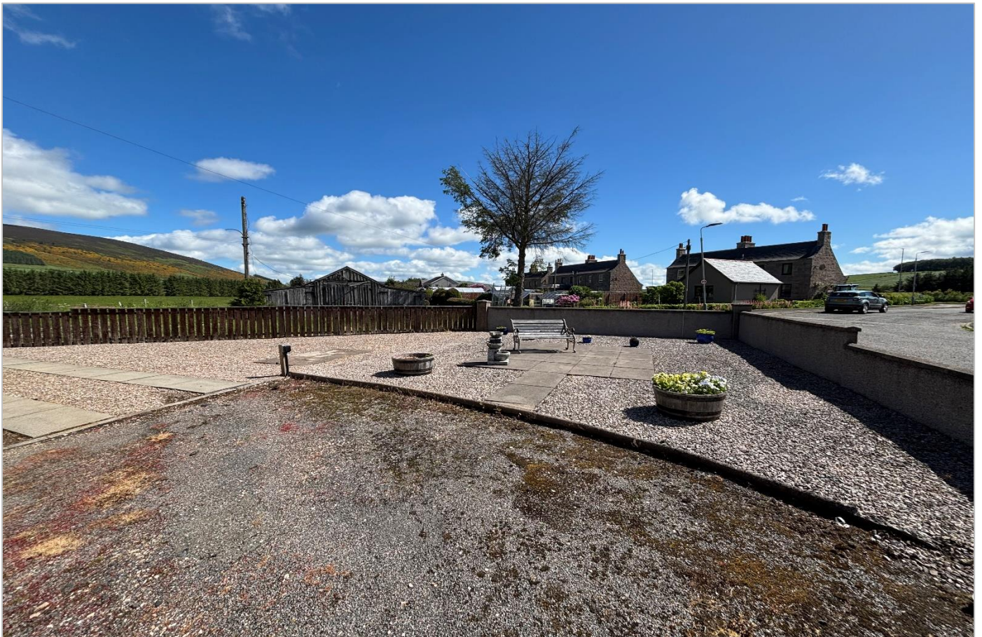
Paved Patio Area
